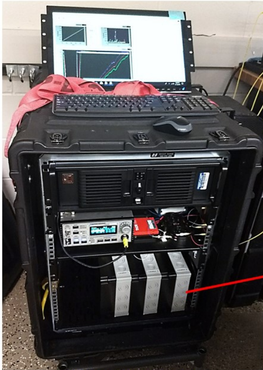
Data acquisition system
